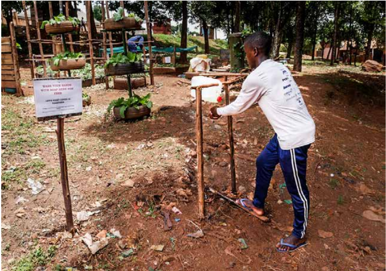
Tippy tap hand washing station installed in Kinawataka community.
